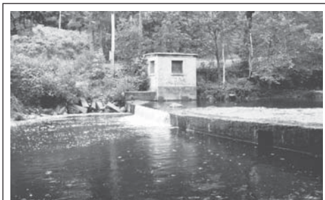
Little River Dam Before
